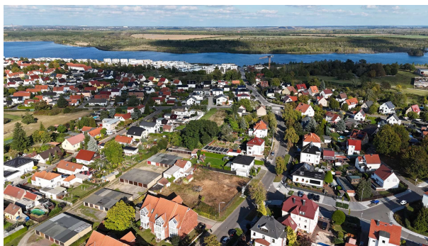
Blick zur Seepromenade
